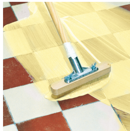
Spread primer over the substrate working in criss-cross method.
