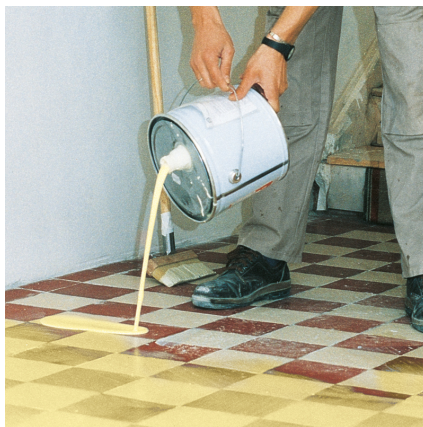
Shake PCI Gisogrund 303 well before use and pour onto the substrate.
