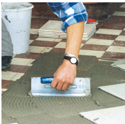
Subsequent top coverings can be applied after approx. 30 to 45 minutes using PCI tile adhesives.
