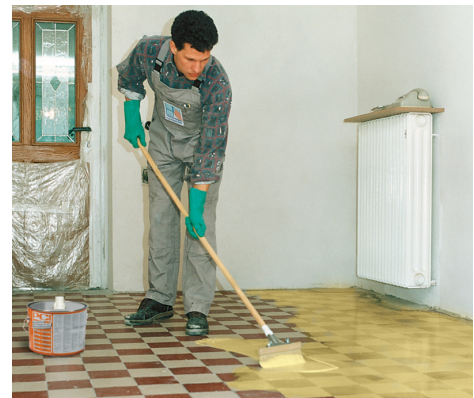
PCI Gisogrund 303 is the reliable primer for laying coverings on ceramic tiles and flagstones.
