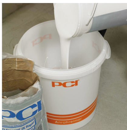
Pour liquid component of PCI Seccoral 2K Rapid in a clean container.
