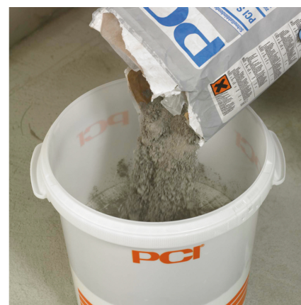
Add PCI Seccoral 2K Rapid powder.
