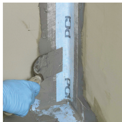
Install PCI Pecitape waterproofing tape in corners.
